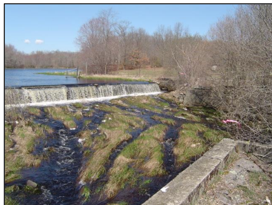
Acushnet Sawmill dam & fishway (2006)
