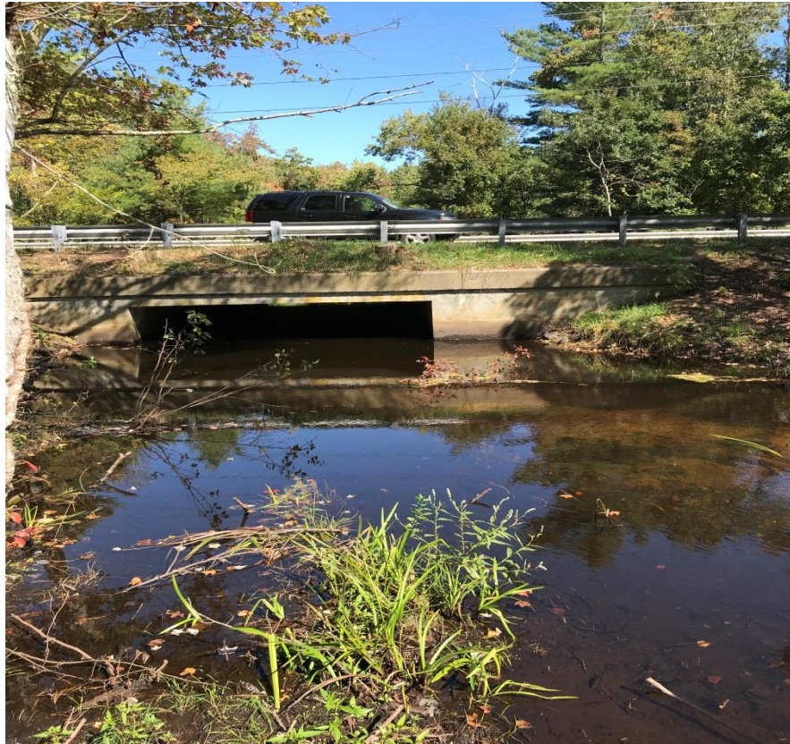
South River, Marshfield – Rt. 139 sand berm removal
