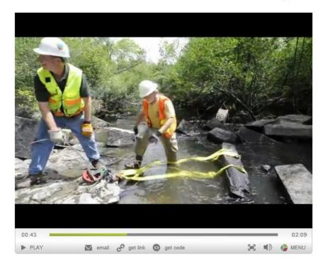
Here's a story about how a cable winch (also known as a grip hoist or come-along) device was used to relocate granite blocks from a collapsed dam to facilitate fish passage. The same technique can be employed to relocate logs in a river to locations where they no longer pose a safety hazard to paddlers.
