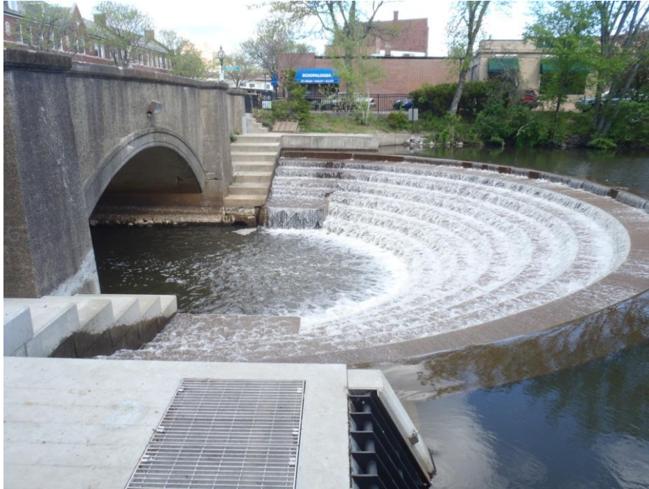
Center Falls Dam, Winchester
