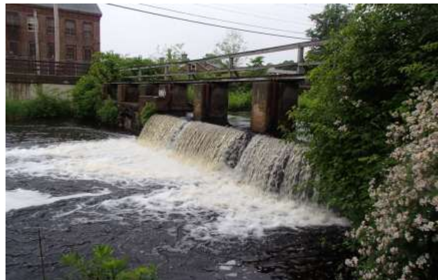
Reed and Barton Dam, Mill River, Taunton
