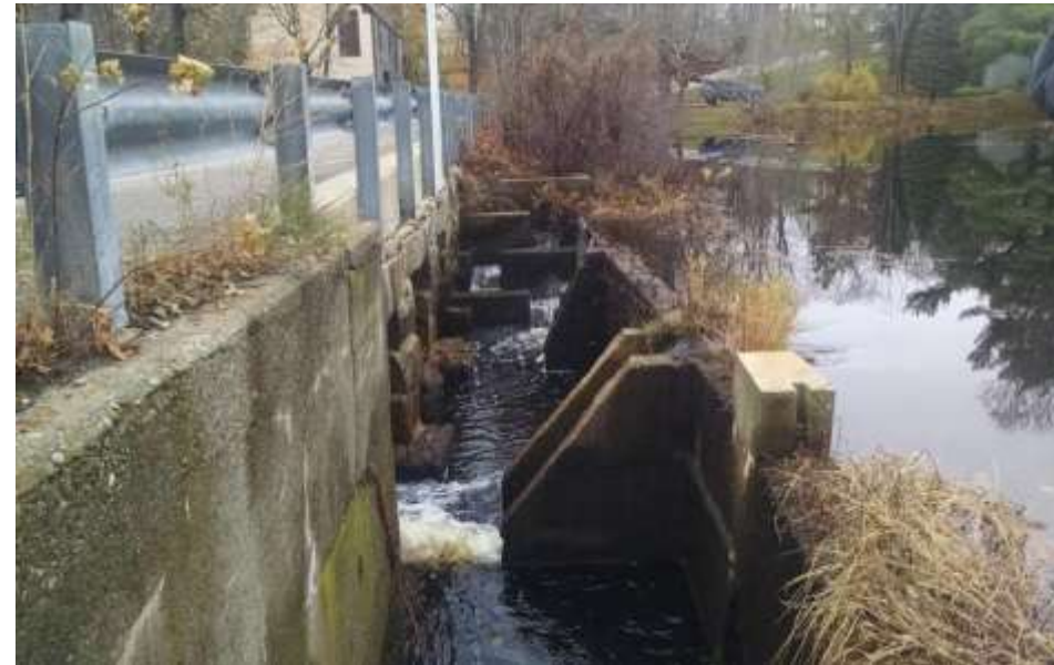
Hunters Pond Dam, Bound Brook, Scituate
