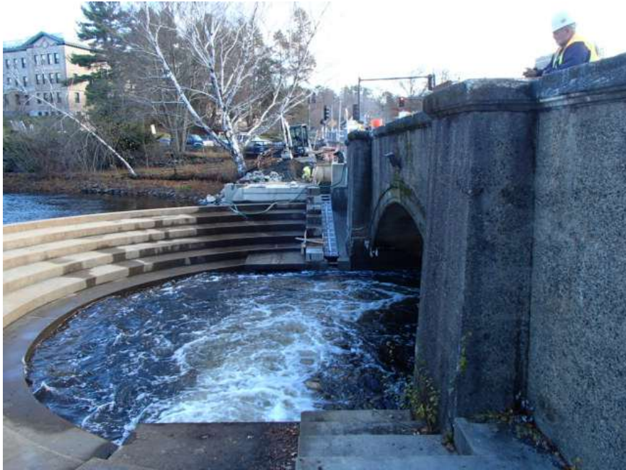
Center Falls Dam, Aberjona River, Winchester
