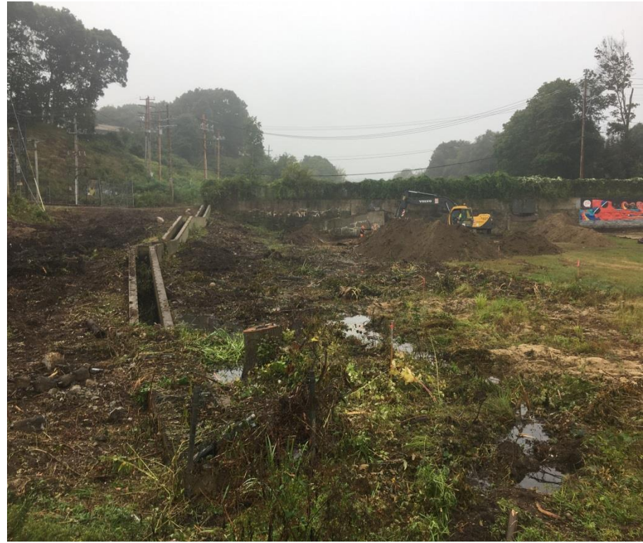
Holmes Dam, Town Brook, Plymouth
