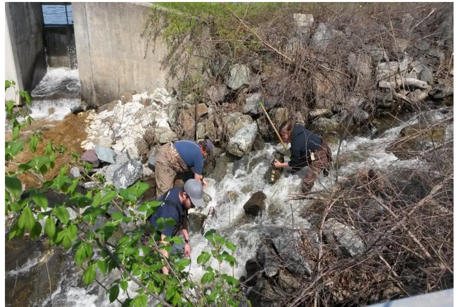
May 2018 spillway ramp adjustments
