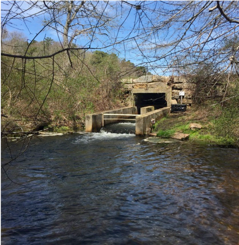
Lower River Culvert
