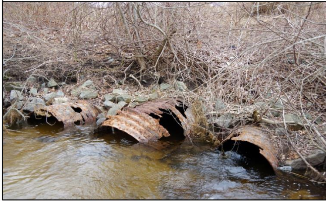
John Parker Road Culvert: design and permitting to replace with a bridge or similar
