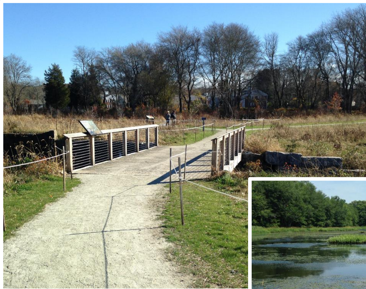
Re-use of bridge with new railings
