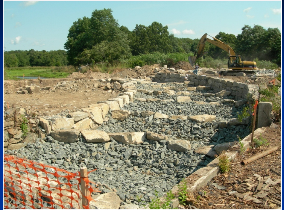
Sawmill Dam fishway construction: July, 2007
